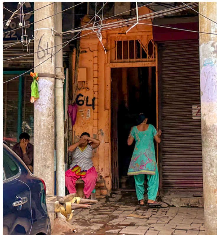
Buildings 59 and 64 on GB Road are where Nepali girls and women are held captive and trafficked.
